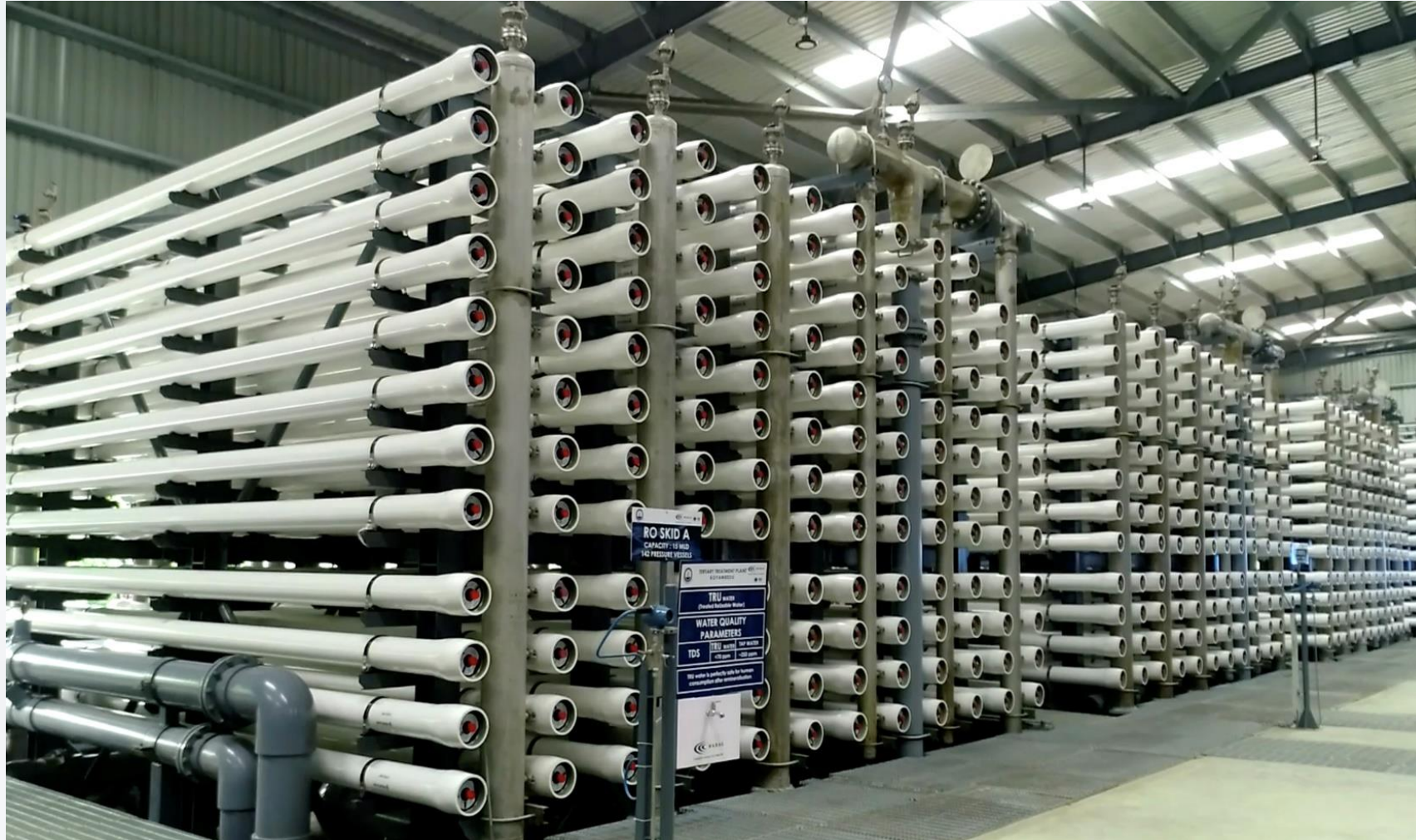
Reverse Osmosis Units (Dow BW30XFR-40034i), Q = 45,000 \text{ m}^3/\text{d} permeate
